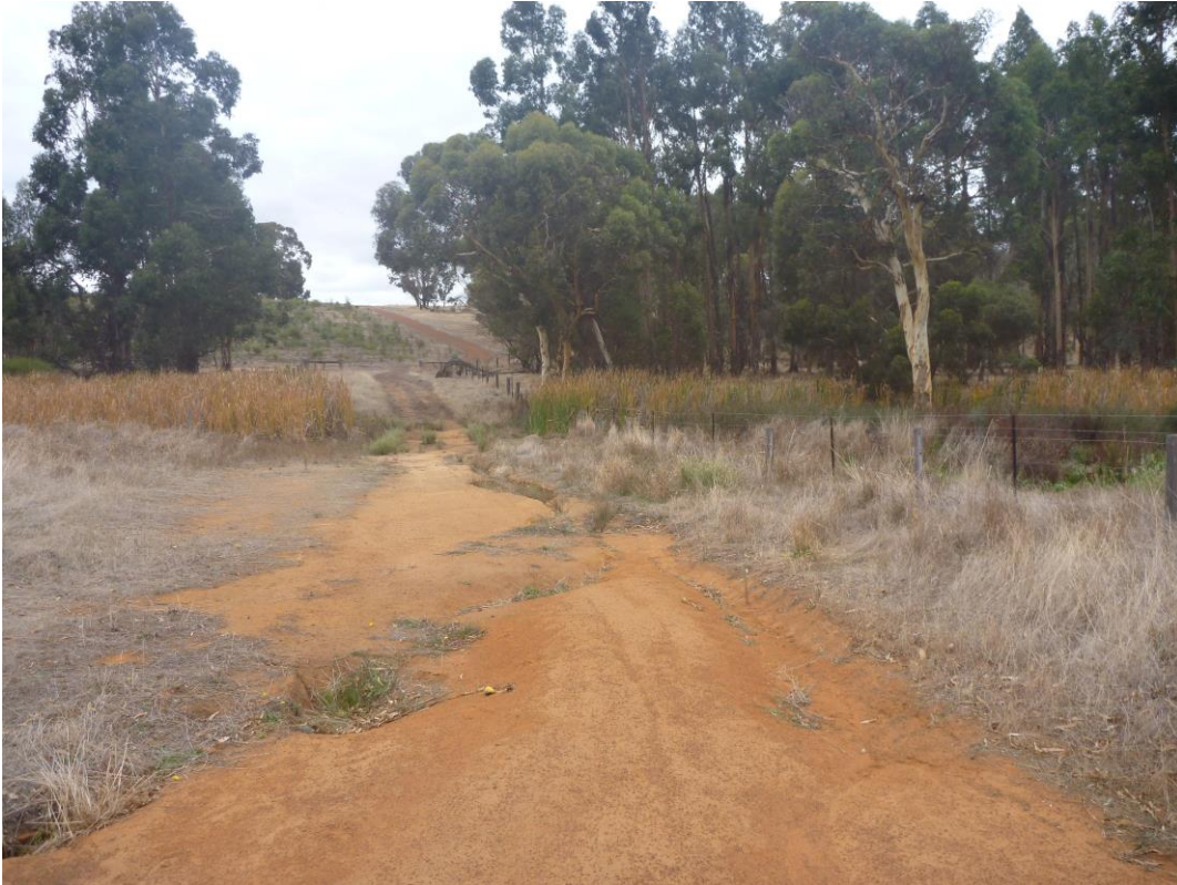
Plate 10: Rill erosion on causeway between north-east paddock and greater restoration area, April 2019
